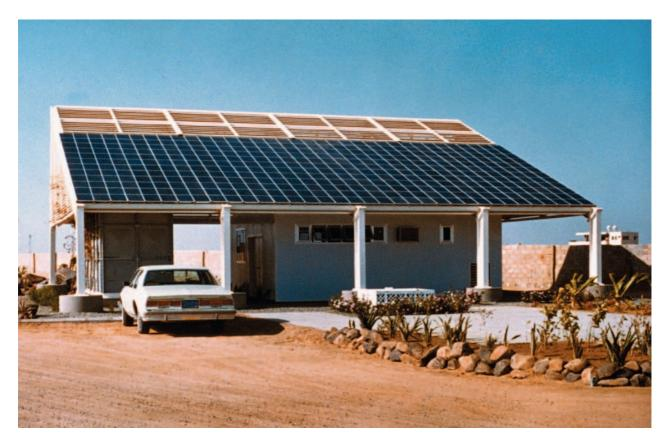
A custom-designed solar powered desalination system in Jeddah, Saudi Arabia. It is composed of 210 photovoltaic modules that supply 8 kilowatts of power (peak) for conversion of highly saline water into fresh drinking water. *Mobil Solar Energy Corporation/Phototake NYC. Reproduced by permission.*
