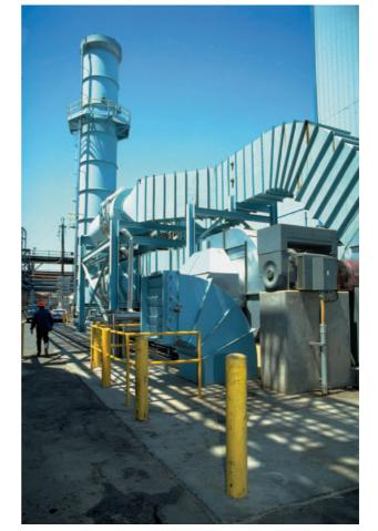
Equipment for the complete recovery and control of air, acids, and oxide emissions. Photograph by Tom Carroll. Phototake NYC. Reproduced by permission.
